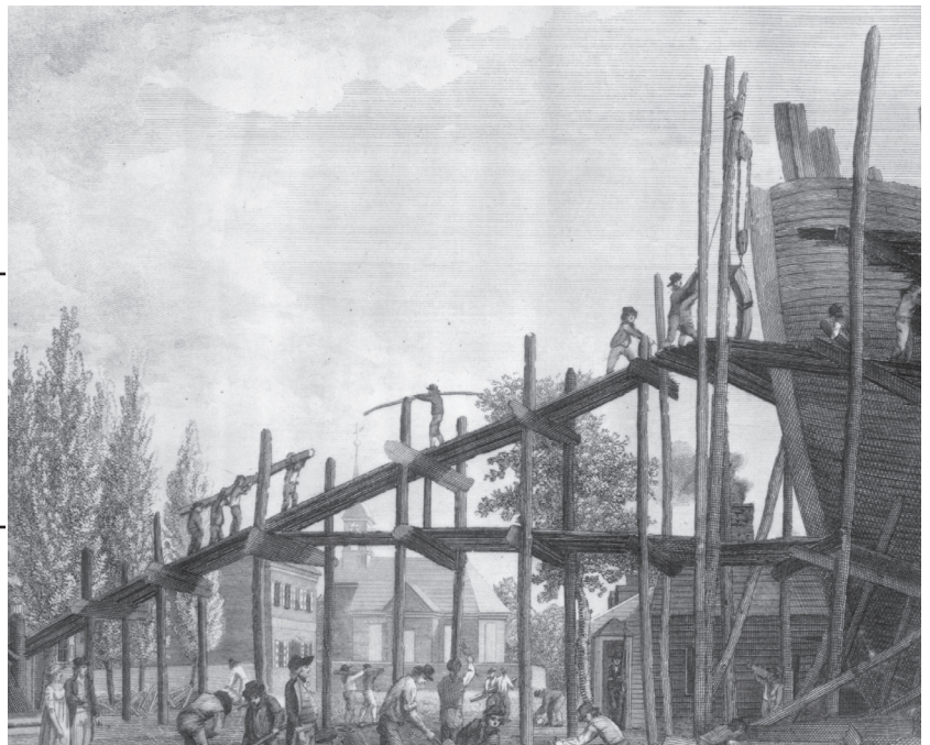
"Preparation for War to Defend Commerce". A late eighteenth-century engraving by William Birch depicted in unusual detail work in a Philadelphia shipyard.
